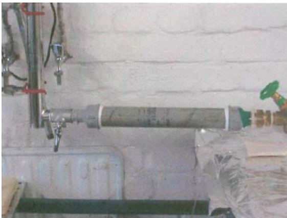
Figure 2: Mixing tank with sampling valve
